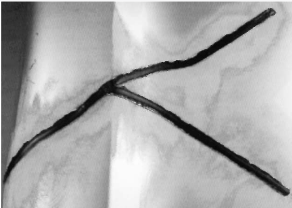
The weld should be a slightly raised, largely smooth, continuous bead.
